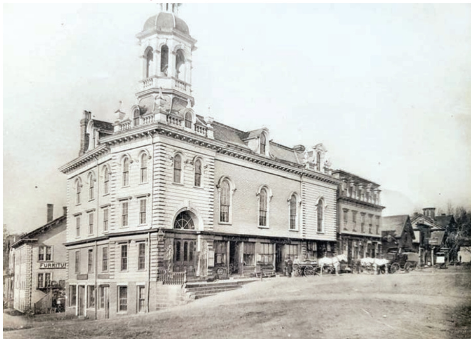
Friends of the North Brookfield Town House plans restoration of the building for use as a civic and cultural center.
